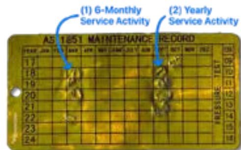
Fig 5: Example of how a servicing plate should be marked
